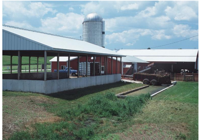
Figure A-6-1. This dry manure stacking facility (at left in photo) is used to store manure until the farmer is ready to treat, transport or apply it. The pictured facility has a roof and concrete walls to prevent manure loss or runoff. Source: NRCS Photo Gallery
