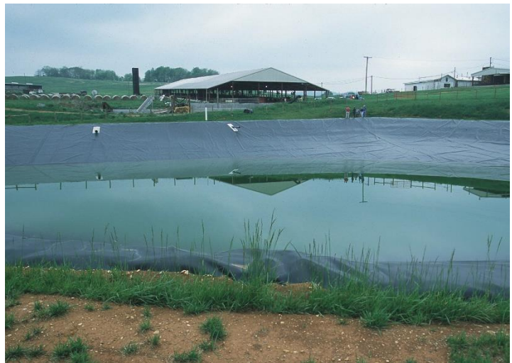
Figure A-6-3. Storage practices come in different shapes and sizes. Storage pits or lagoons are used for liquid manure such as dairy cow or swine manure. Pictured is a lagoon in Virginia. Source: NRCS Photo Gallery
