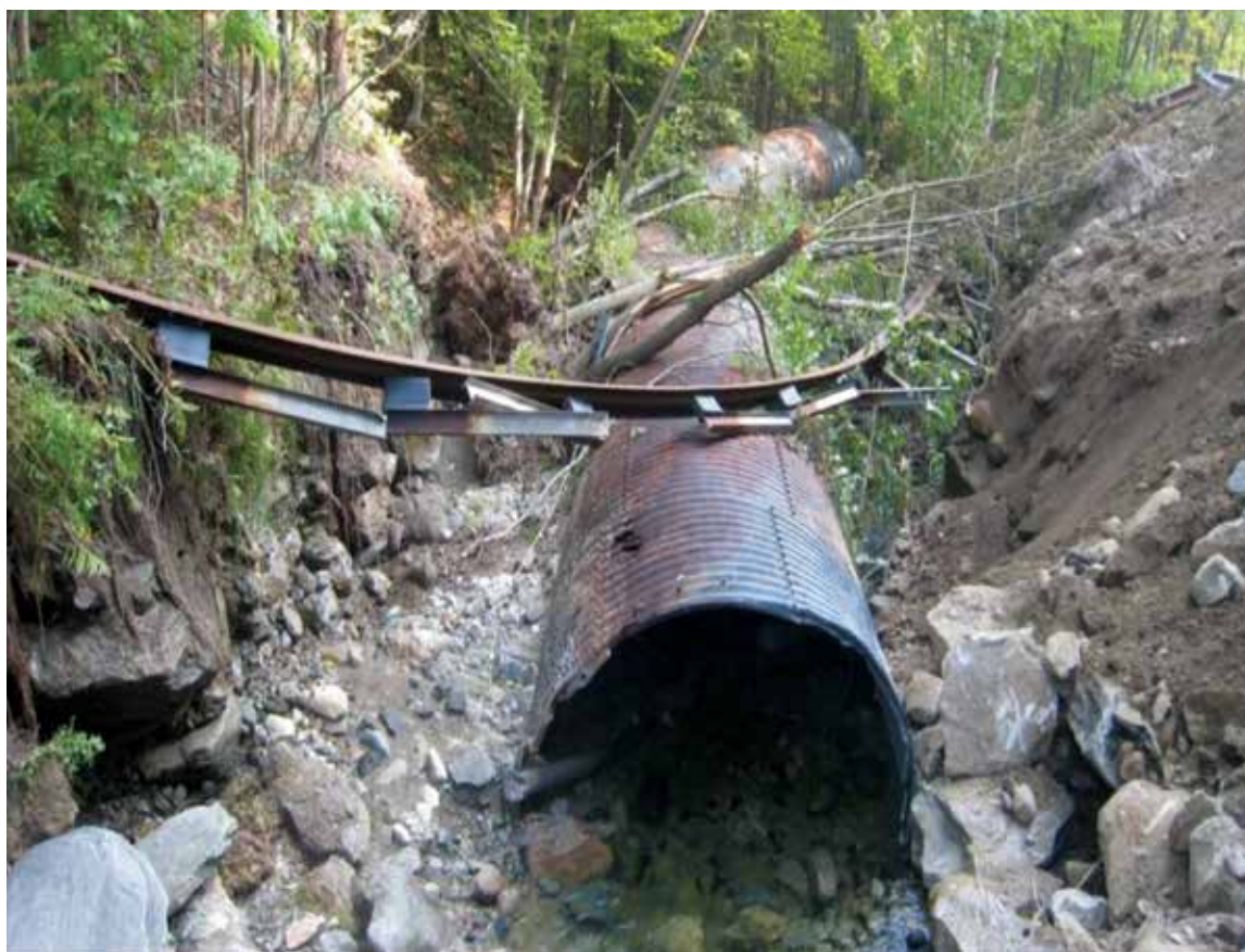
Figure 1. Road failure at a 3-m culvert placed within a 6-m bankfull width stream, Green Mountain National Forest. Photo credit: Dan McKinley, Green Mountain National Forest.
