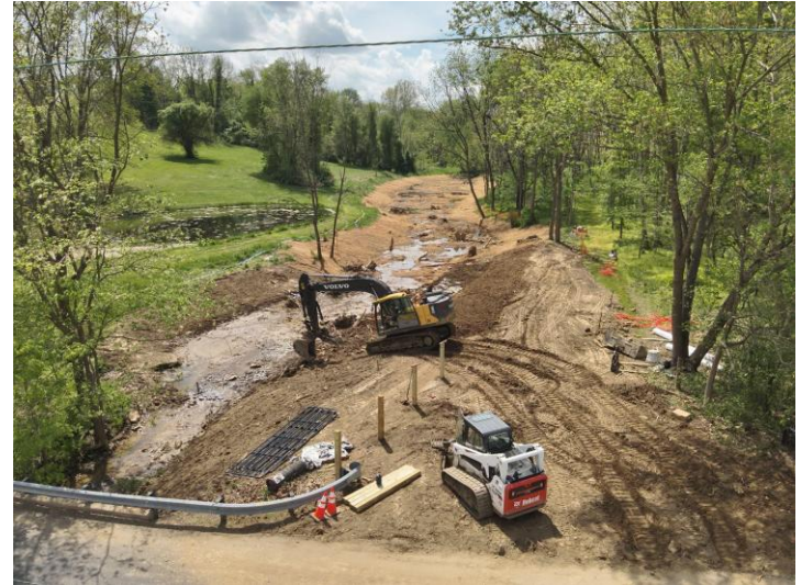
Machinery working during the construction of a restoration in Millersville, Pennsylvania.
