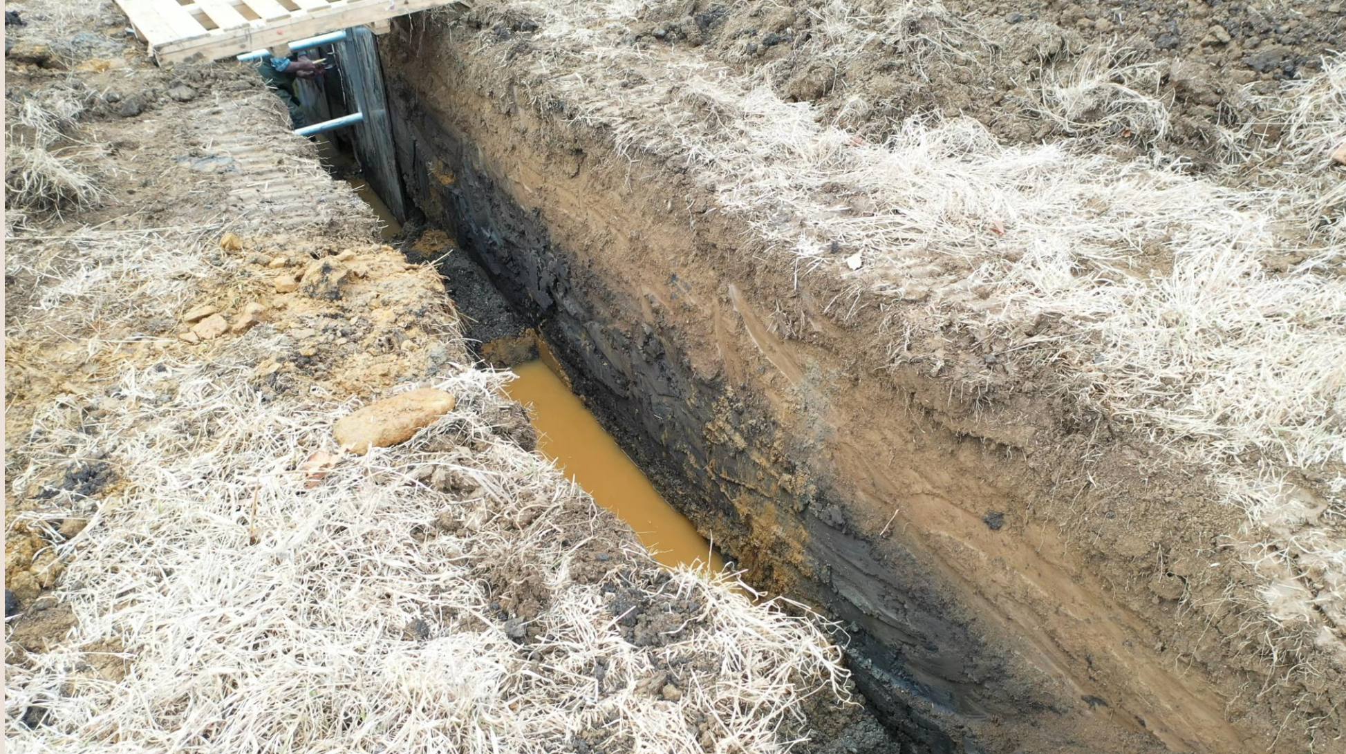
Woodcrest Villa Trench Site 2/13/23
