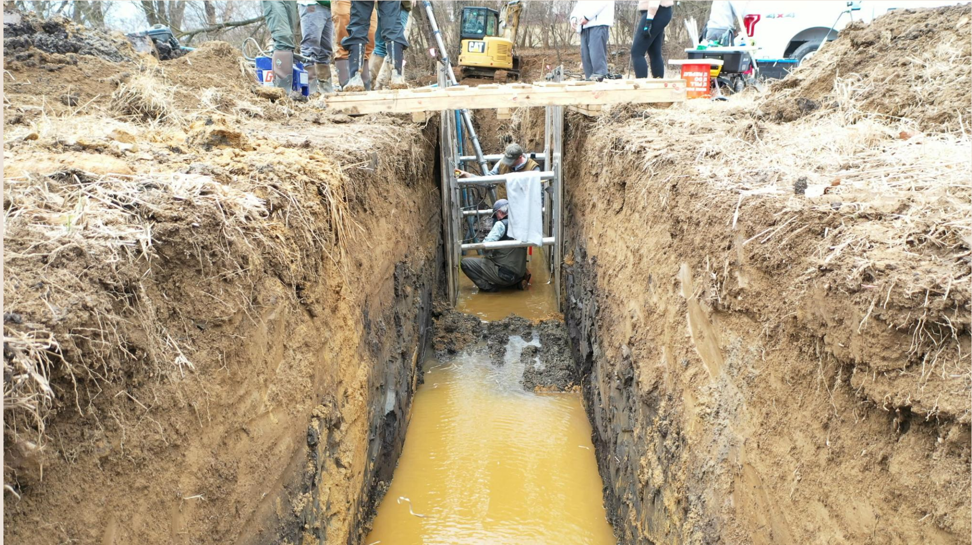
Woodcrest Villa Trench Site 2/13/23
